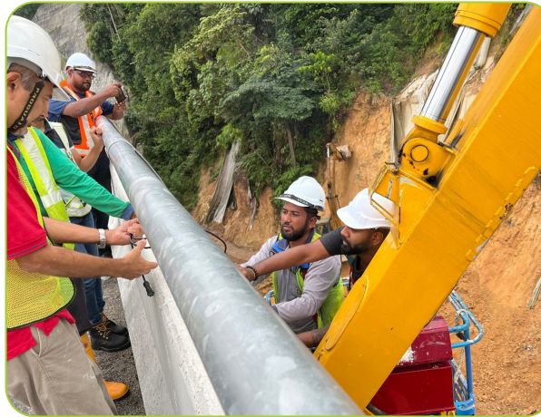
Installation of the Gateway required the use of a skylift to mount the unit onto the bridge wall
