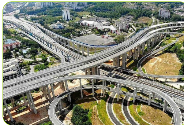
The Sungai Besi-Ulu Kelang Expressway (SUKE)
